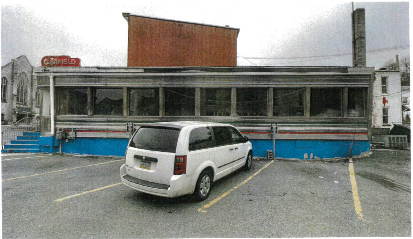
Side view of 402 W. West Market Street Diner
